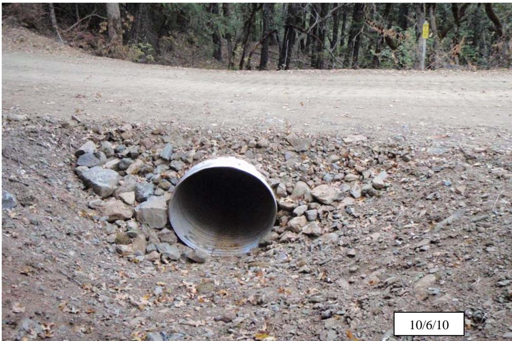
**Photo 2b.** Cecilville/Taylor Road #1, site #42, similar view as above, after implementation. The channel has been excavated with 2:1 side slopes above the crossing, and a 36 in. diameter  $\times$  40 ft long culvert installed. Rock armor has been placed along the inboard fill for fillslope protection.
