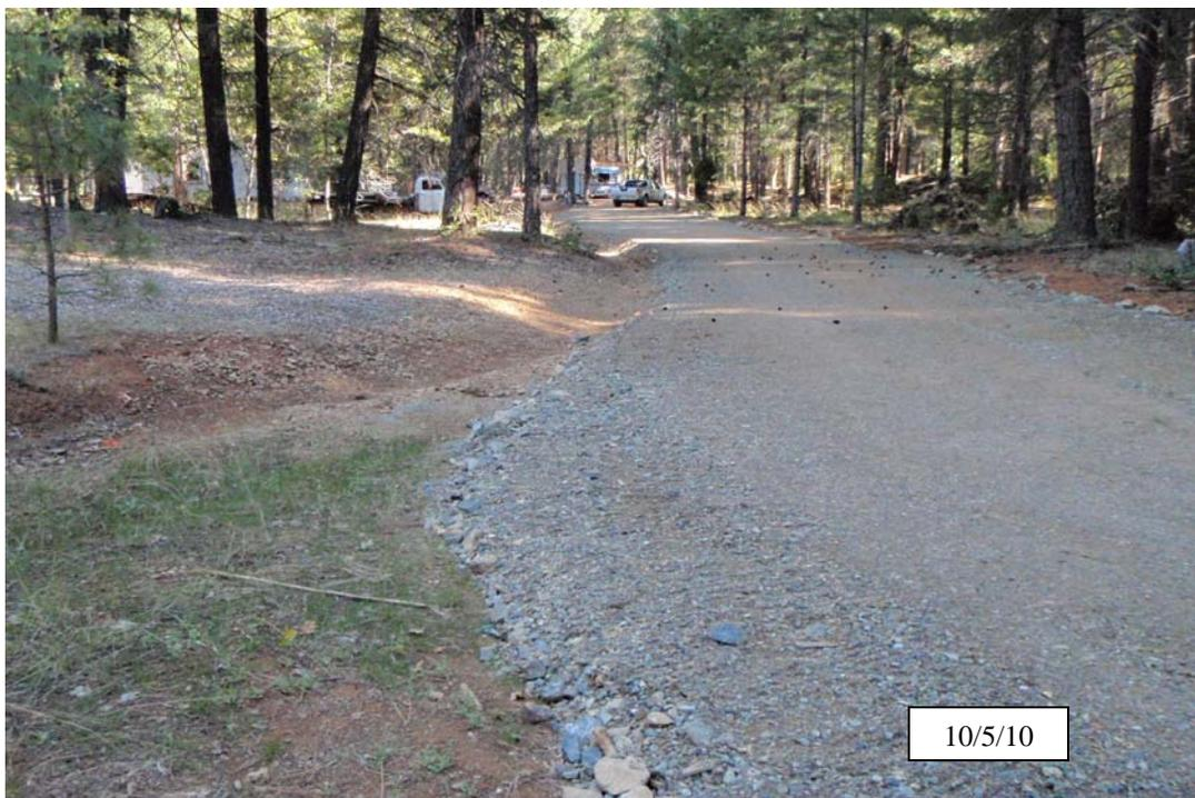
**Photo 5b.** Finley Camp Road #1, similar view as above, after implementation. The road has been widened and road rock was applied. The inboard ditch (on left) was widened and deepened.
