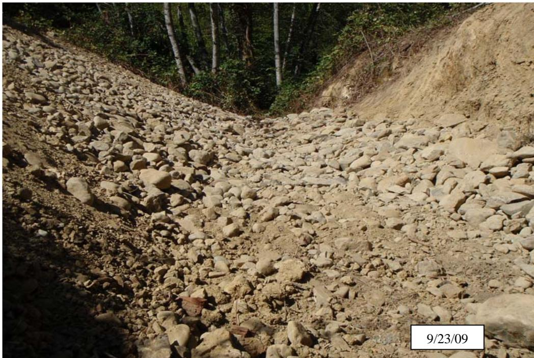
**Photo 1b.** Bloomer Mine Spur #1 Road, site #3, same view as above, after implementation. The stream crossing has been decommissioned with a 6' channel bottom width and 2:1 sideslopes, except on the left bank where bedrock is exposed. Bare soil areas were mulched with straw after the photo was taken.
