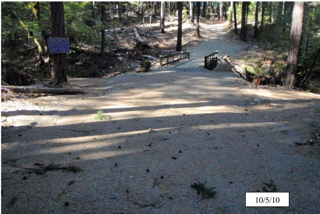
**Photo 6b.** Finley Camp Road #2, site #36, similar view as above, after implementation. View from the right road approach, looking across the new bridge crossing of the Class I stream. Both road approaches had road rock applied.
