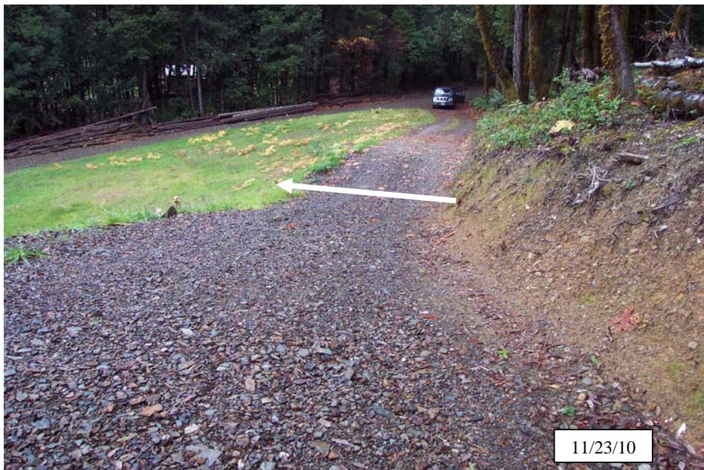
**Photo 12b.** Butler Flat loop Road, rolling dip # 3.1 location (arrow), after implementation.
