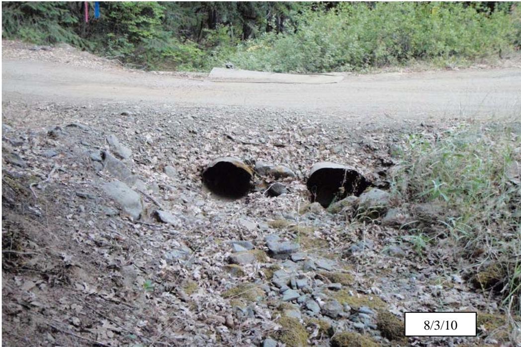
**Photo 2a.** Cecilville/Taylor Road #1, site #42, before implementation. View from the top of the site, looking downstream at a crossing of a Class III stream. Prior to treatment, there were two, mostly plugged and rusted out culverts at this site. Note the plywood on the outside edge of the road.
